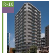
R-10 KDX Residence Kikusui Yojo
