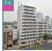
T-5 KDX Bunkyo Sengoku Residence
