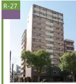
R-27 KDX Residence Sannomiya
