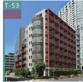
T-53 KDX Residence Shinagawa Seaside
